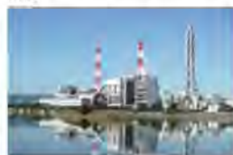
1. Trailblazer. The 250-MW IGCC demonstration plant at Nakoso, Japan, owned by Mitsubishi-Hitachi Power Systems, has been operating successfully since 2007. Courtesy: MHPS.
