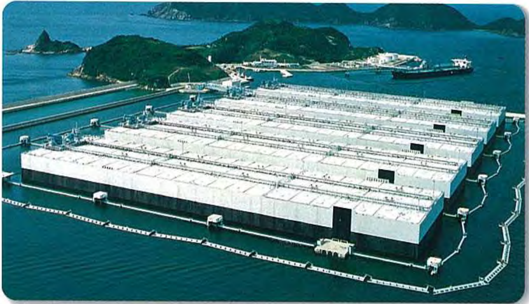
上五島石油備蓄基地 Kami-goto floating crude oil storage facility
